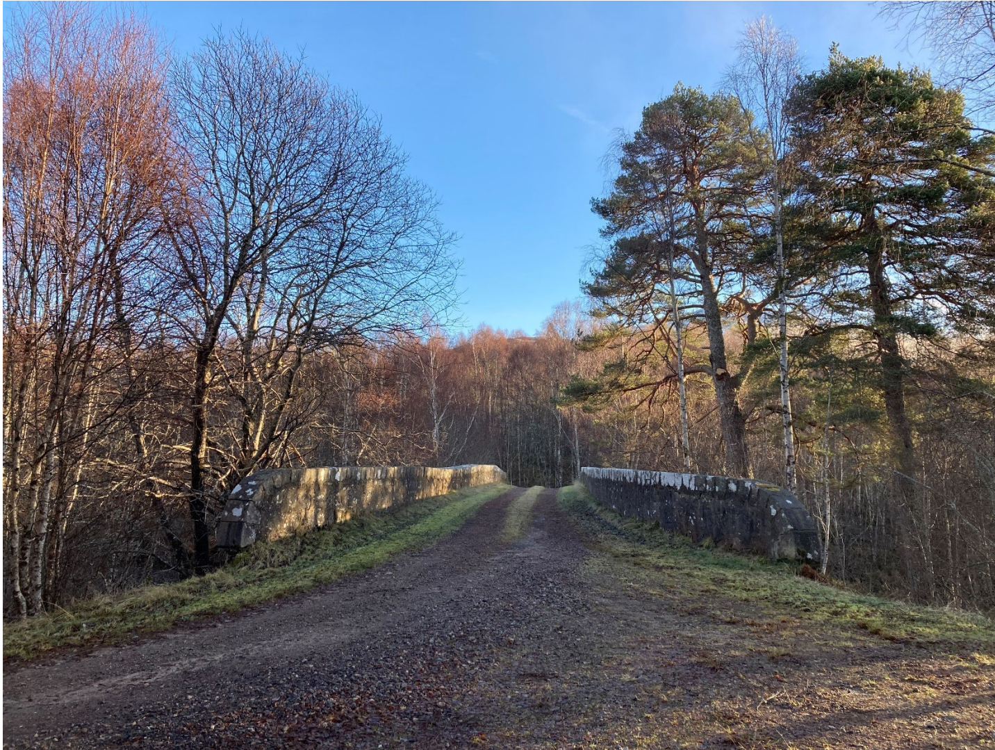
Photograph 5: Listed Bridge at Ceanacroc (looking S/SE)
