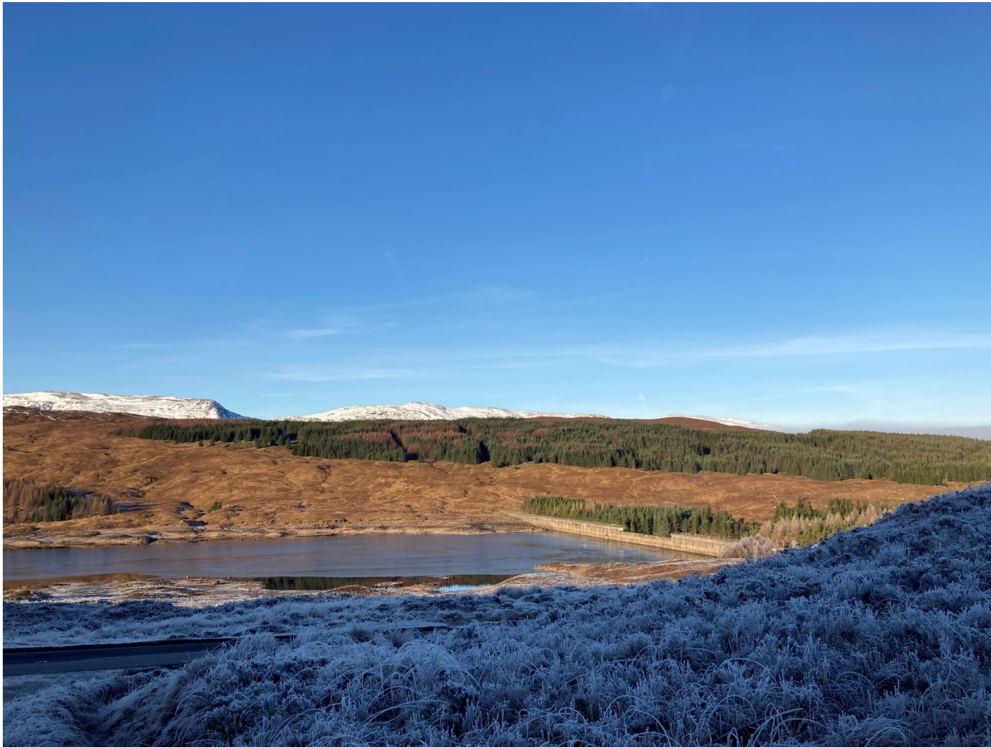
Photograph 9: View towards Loyne Bridge and associated dam from access gate (looking W/NW)
